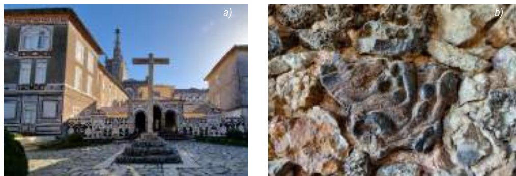
Fig 1. (a) early 17th century embrechado decoration on the western façade of the Convento de Santa Cruz do Bussaco. The dark component is provided by slag from bloomery iron smelting. (b) detail of embrechado decoration inside the entrance hall of the Convento, showing a block of tapped bloomery iron smelting slag. The chemistry of the slag is compatible with the smelting of iron ore hosted by the Ordovician Porto de Santa Ana Formation, as seen at the ancient smelting sites such as Vinha da Leira Má (Louredo) and 'Pedras Negras' (Vicariça).
