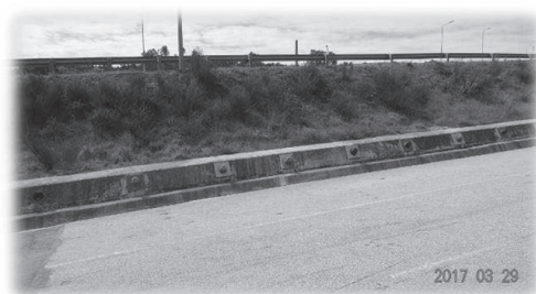
Anchored retaining beam and anchor pressure gauge.
