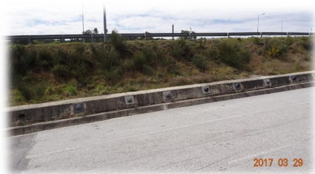
Anchored retaining beam and anchor pressure gauge.
